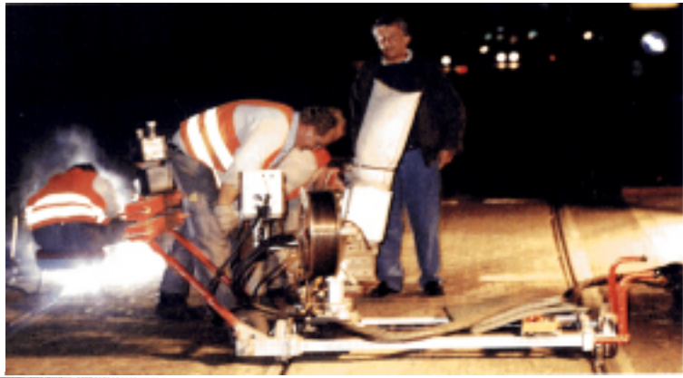
Figure 7: Two welding processes in night-time performance comparison on a rail curve
