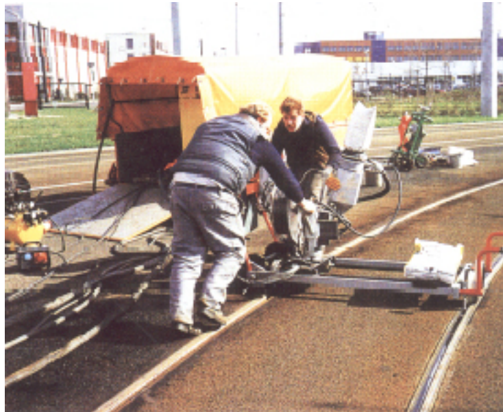
Figure 3: Manual positioning of the automatic welding machine with a disengaged drive unit
