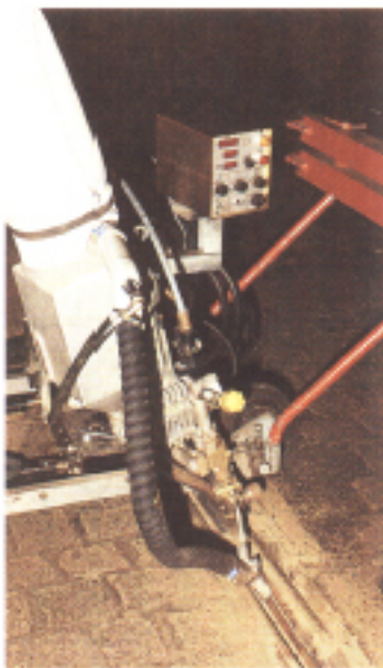
Figure 2. A6S-automatic welding machine in operation
